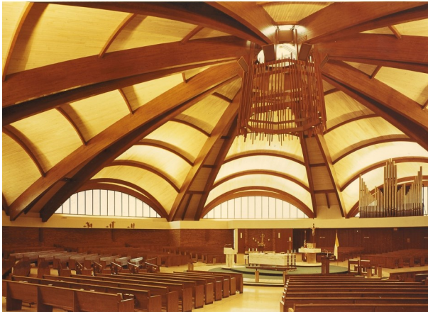
Arches made in Peshtigo for roof supports of Good Hope Catholic Church in Milwaukee, WI
